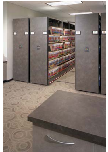
After – Added Rails For Floor Loading
