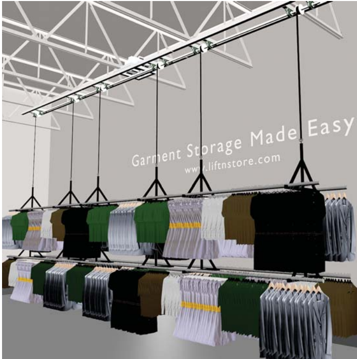
Shown above is the LiftNStore® Overhead Quad Garment Lift, model LG-1033. The footprint is 24 feet long and features 96 feet of open hang bar space.
