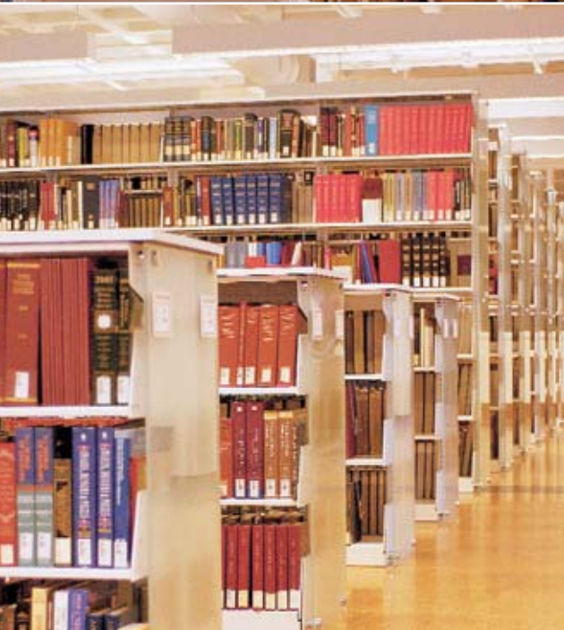
Extra-tall Spacesaver mobile and stationary shelving optimize space in the Special Collections area. Reference shelving features custom glass end-panels.
